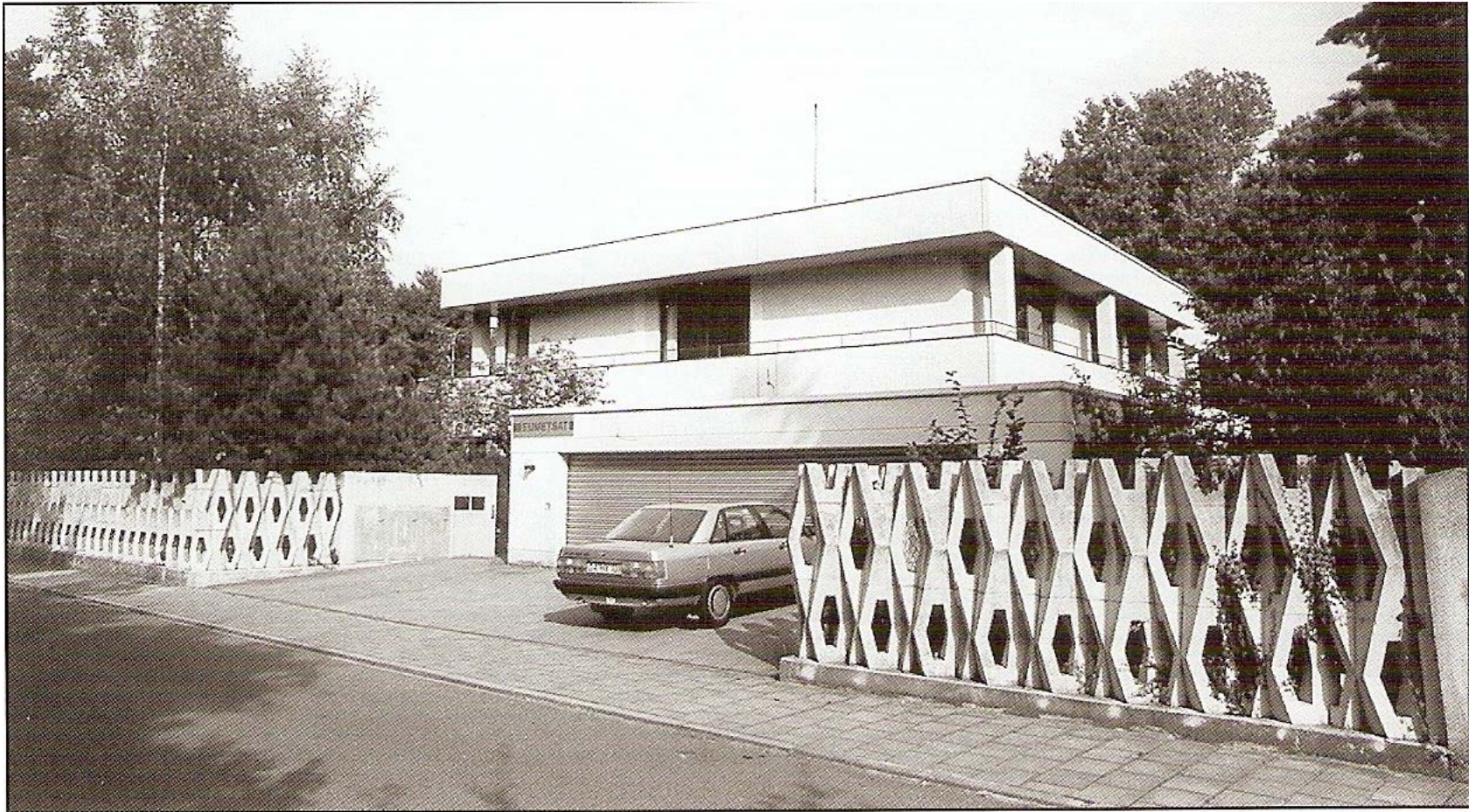
Temporary headquarters, Am Elfengrund, Darmstadt-Eberstadt
